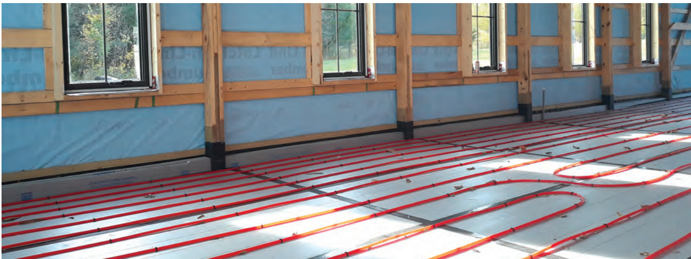
A barndo in progress in Milaca, Minnesota, featuring Plasti-Sleeve, Plasti-Skirt, and in-floor heat. PHOTO COURTESY OF PLASTI-SLEEVE
