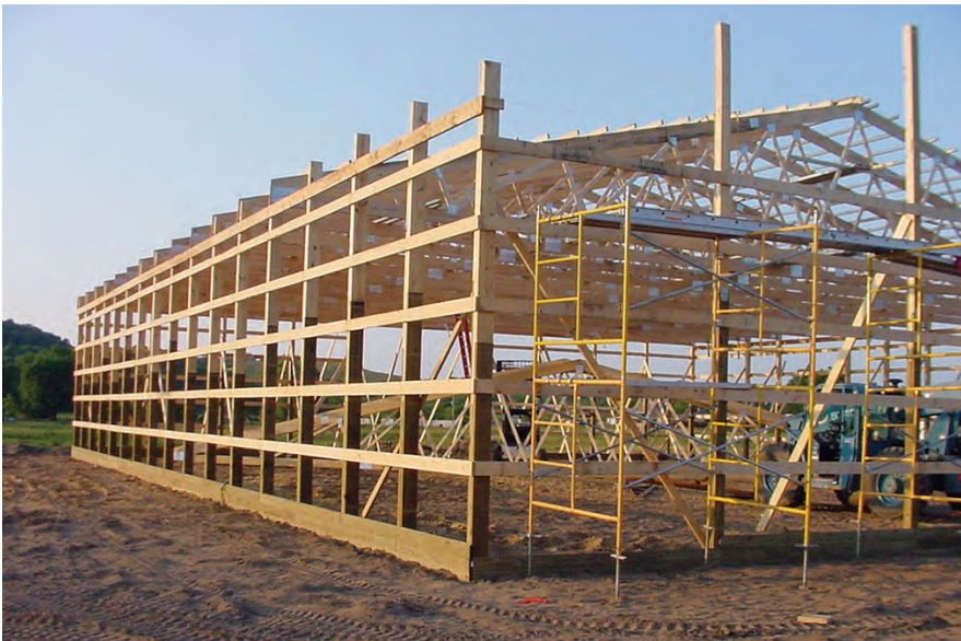
Interior bracing.
