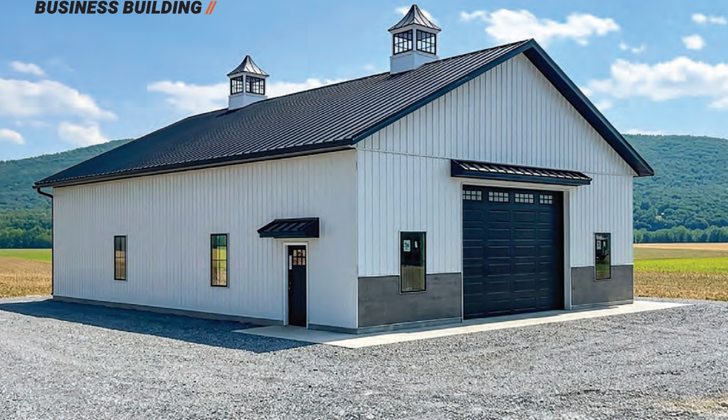
PHOTOS COURTESY OF WHITETAIL CONSTRUCTION
