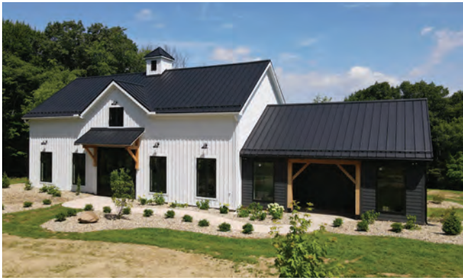
Board and batten siding with overhangs definitely says “residential.” IMAGE COURTESY OF METAL EXTERIORS
