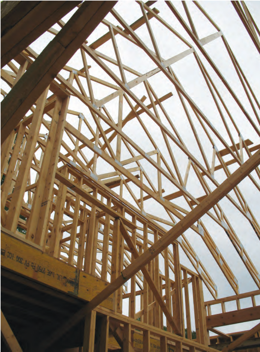
Parallel chord bracing.
