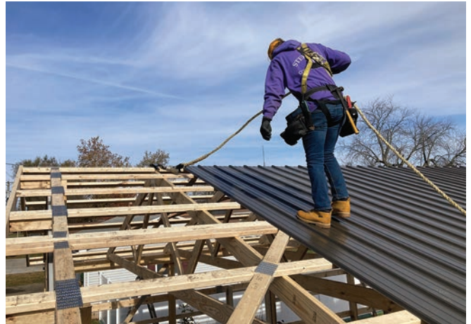
Fall protection systems should be used at every stage of installation.
