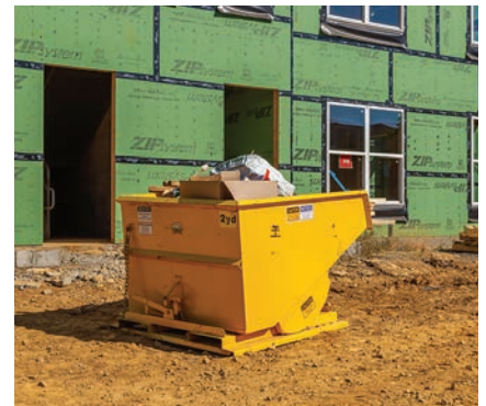
Set up the hopper close to work in progress.
