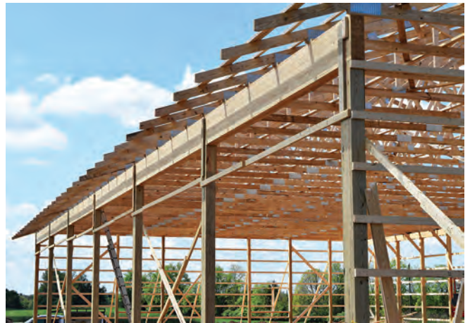
Booth 536: Rigidply Rafters Glulam Posts.
