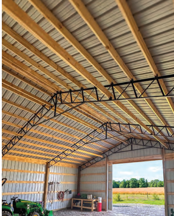
COURTESY OF TROYER POST BUILDINGS
