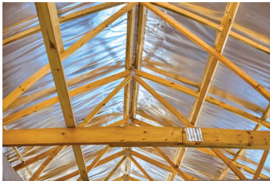
COURTESY OF TROYER POST BUILDINGS
