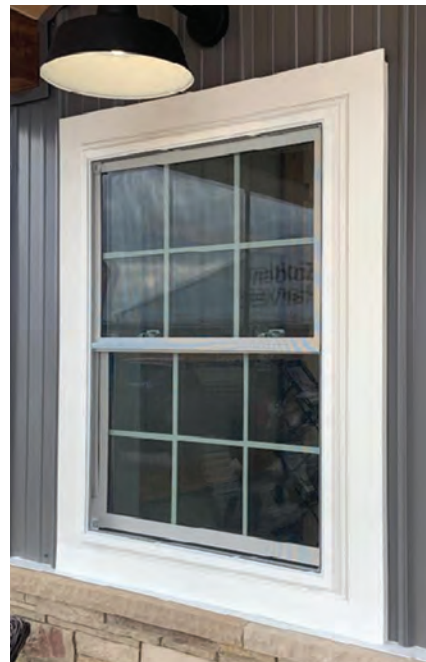
Harmony vinyl double hung with grids in the airspace and nail fin. PHOTO COURTESY OF AJ MANUFACTURING
