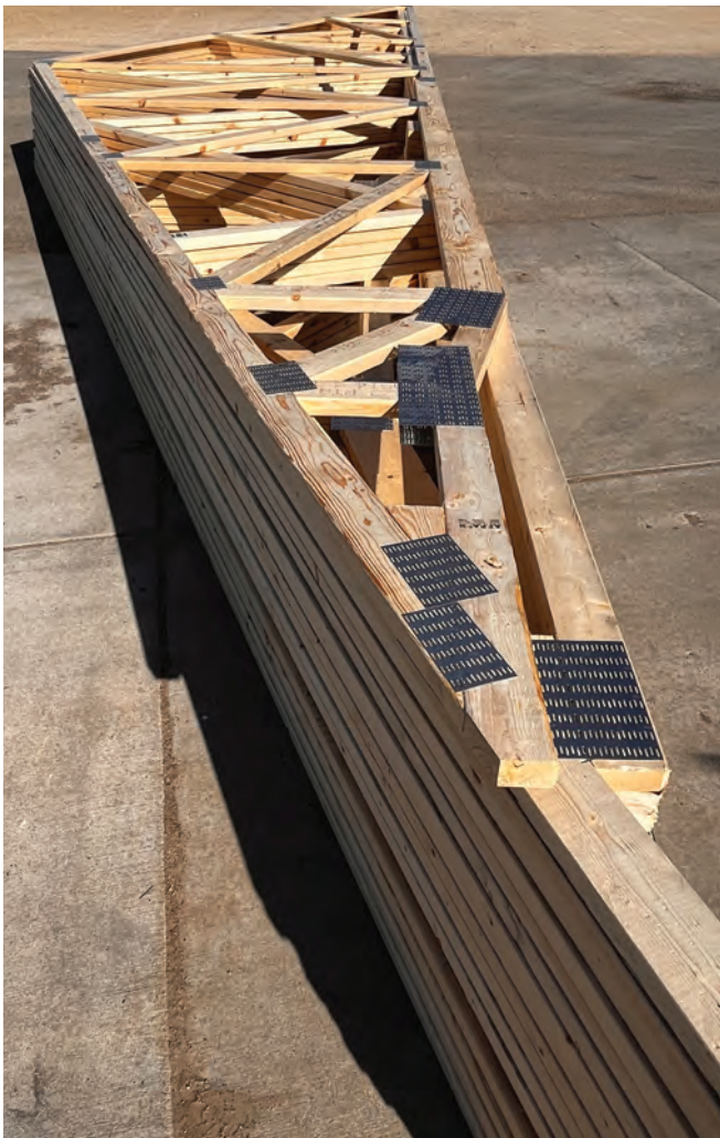
Deferred submittals, like truss packages, must be reviewed and approved before installation, placing additional responsibility on both the framing contractor and owner to ensure compliance. PHOTO COURTESY OF SBCA.
