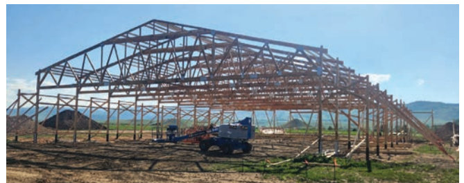
Framing system intact. ALL IMAGES COURTESY OF HANSEN POLE BUILDINGS
