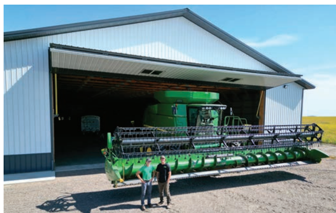
Bifold doors open outside the building so they don't reduce headroom.
