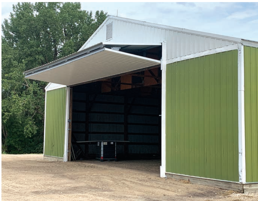
Bi-fold doors do not obscure the building's opening, allowing equipment to use the full height and width of the doorway when entering or exiting. PHOTOS COURTESY OF MIDLAND DOOR SOLUTIONS
