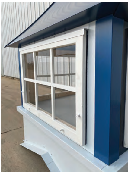
Cupola with new Cupola Access Window.
