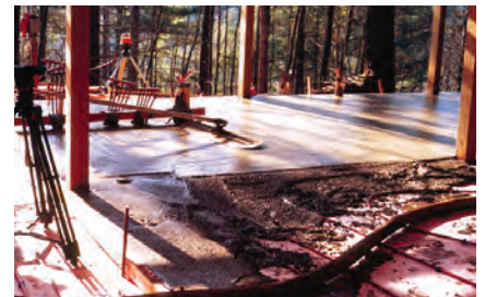
Before the warmth: If the boiler is the heart of a hydronic radiant system, the PEX tubing represents the blood veins. These tubes are strategically spaced throughout a building's floor plan, spaced closer together where more heat will be needed, further apart in other areas. The pipes are then covered with concrete or a gyp-crete alternative, which provides thermal mass.
