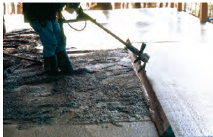
Before the warmth: If the boiler is the heart of a hydronic radiant system, the PEX tubing represents the blood veins. These tubes are strategically spaced throughout a building's floor plan, spaced closer together where more heat will be needed, further apart in other areas. The pipes are then covered with concrete or a gyp-crete alternative, which provides thermal mass.
