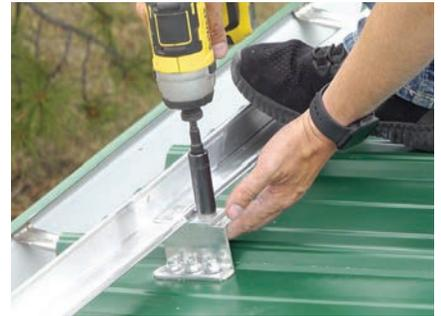
VersaBracket is a bottom-fixed, metal roof bracket designed for mounting ColorGard, solar PV, and other utility mountings to exposed fastened profiles. VersaBracket features a 1" mounting slot on the top flange for adjustability and fastens through the roof, into the deck or structure. Factory-applied butyl sealant ensures speedy installation and lifetime performance.
