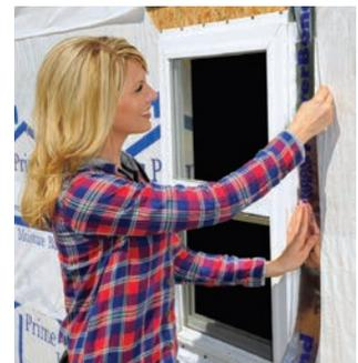
Extend your building season with WindowWrap PowerBond adhesive system, which aggressively adheres in cold weather down to 25° F, while remaining stable at elevated temperatures. It features a flex option for sill pan flashing and curved openings, self-seals around common fasteners, is more economical than butyl-based products, and is made in the USA.
