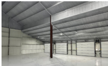
Building using Firestable.
