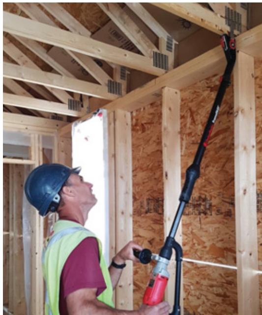
FastenMaster FrameFAST is a better way to make critical connections along the continuous load path, FastenMaster says, citing "One screw, one tool, and three interchangeable heads replace a variety of clips."
