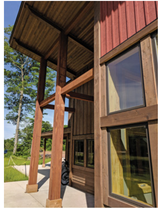
Glulam columns used for architectural exposed purposes on the Berkie Trailhead structure near Cable, Wis. (PHOTO COURTESY OF TIMBER TECHNOLOGIES)
