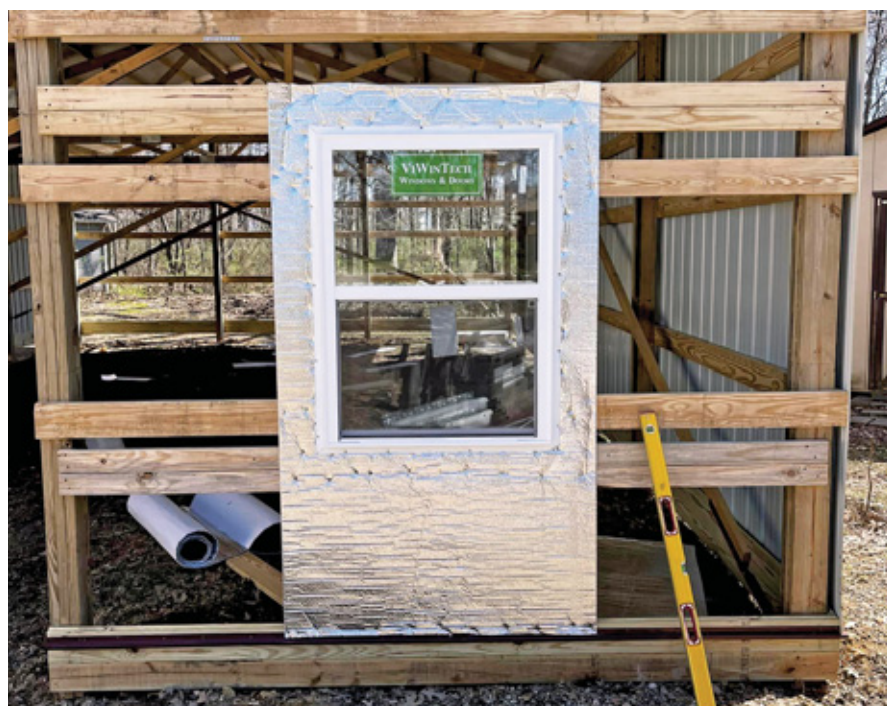
Builder Kevin Delay's company orders windows with integral J-channels and overlaps the trim with a reflective radiant barrier.
