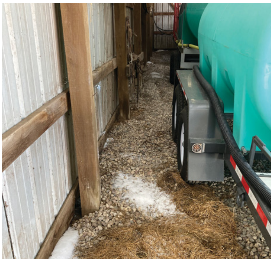
This building has had gravel added after the initial build.
