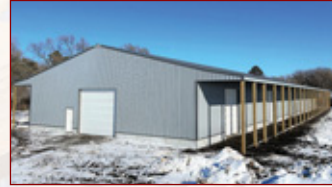
Livestock Sheep Facility: Critel Buildings
