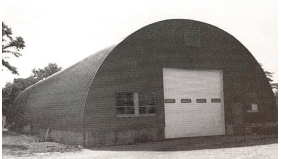
The finished product transformed an “about to be condemned building” into an eye-pleasing structure that is a valuable part of the local industrial park.
