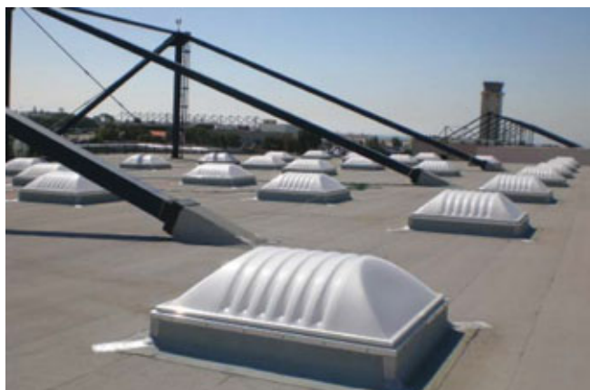
A typical polycarbonate skylight used for toplighting commercial spaces is depicted above. (COURTESY OF ACUITY BRANDS)
