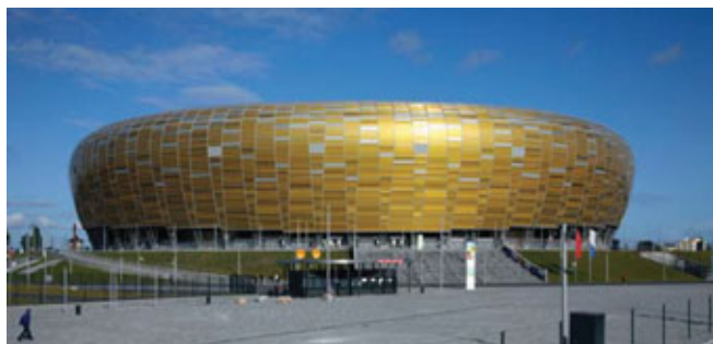
The PGE Arena Gdansk soccer stadium in Danzig, Poland, is clad with 45,000 square meters of multicolored, multiwall polycarbonate sheet.
