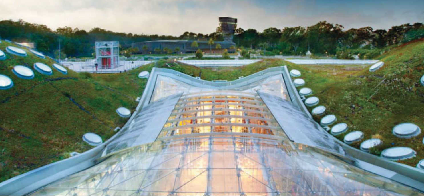
The California Academy of Science Building in San Francisco, California, USA uses coated polycarbonate sheet for the operable section of the building's roof.
