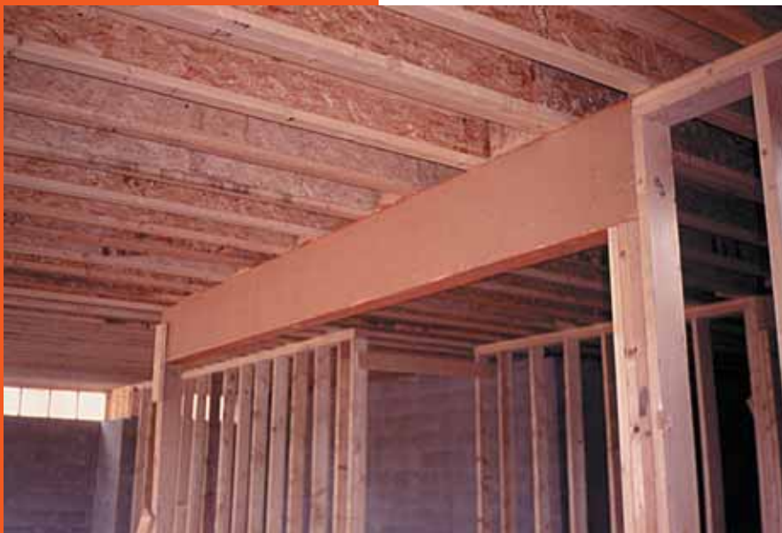
Depending on the load requirements, laminated veneer lumber (LVL) can be used interchangeably with glulam beams.
