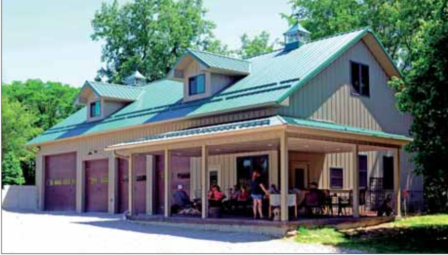
(Above) The residential market is growing as more consumers are learning about the benefits of post-frame construction. PHOTO COURTESY OF WICK BUILDINGS
