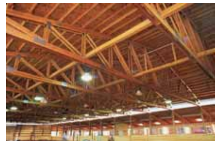
Post-frame structures offer builders many opportunities to use engineered lumber. PHOTOS BY APA-THE ENGINEERED WOOD ASSOCIATION
