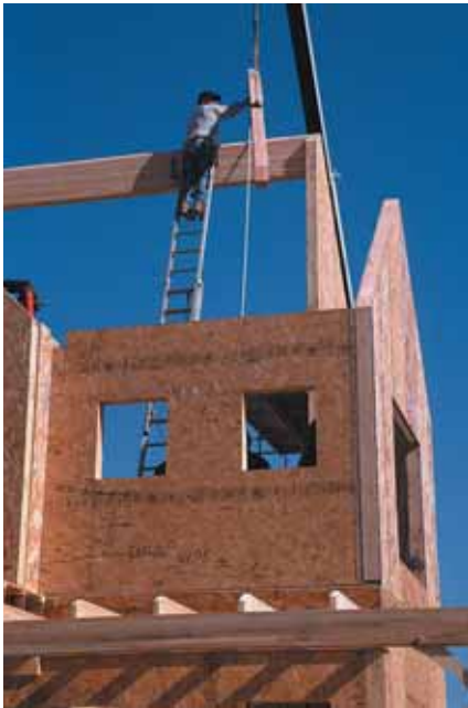
A glulam ridge beam supports SIP (structural insulated panel) roof panels. NOTE: THIS PICTURE WAS ORIGINALLY PUBLISHED 20 YEARS AGO. FRAME BUILDING NEWS ADVISES ALL OSHA-REQUIRED SAFETY EQUIPMENT BE USED.
