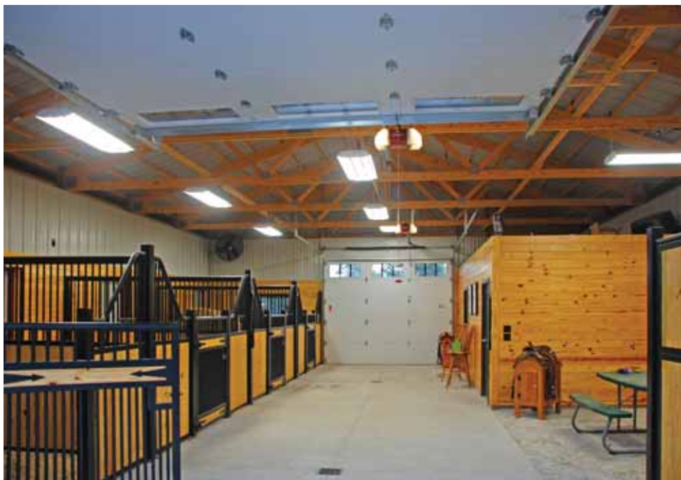
Large roll-up doors on both ends, eave and ridge vents are all part of the passive ventilation system in this horse barn. Stall fans and grilled stalls also help facilitate the distribution of fresh air. PHOTOS COURTESY OF WICK BUILDINGS.
