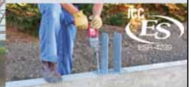
Sturdi-Wall™ Brackets Drill set for cured foundations
