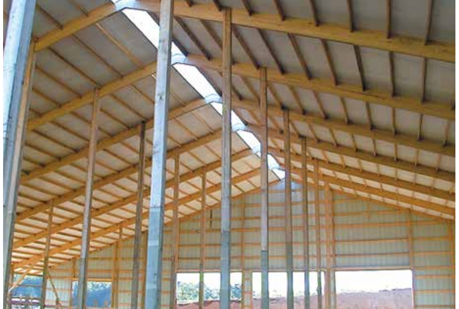
Installing the foil-faced insulation below the metal roof panels and above the purlins resulting in an effective thermal break. The foil faces the metal panel, which reflects the heat and prevents significant heat gain. Photo courtesy of rFOIL Covertch.
