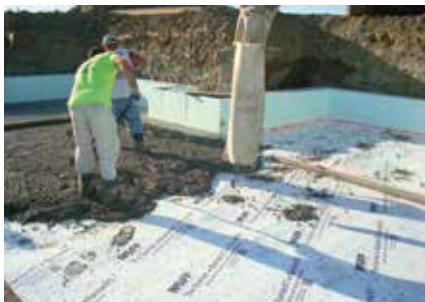
An underslab barrier prevents moisture intrusion up through the concrete and unwanted heat transfer. In this case, it also stops radon gas from permeating the concrete. Shown: The Barrier by NOFP. Photo courtesy NOFP, Inc.
