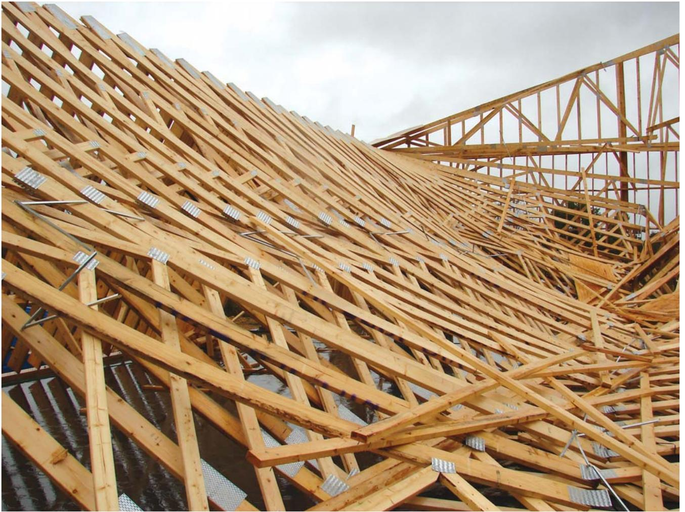
the production and delivery of a replacement truss. The sooner the CM is contacted, the less disruptive the remedy will be to the installation process.
