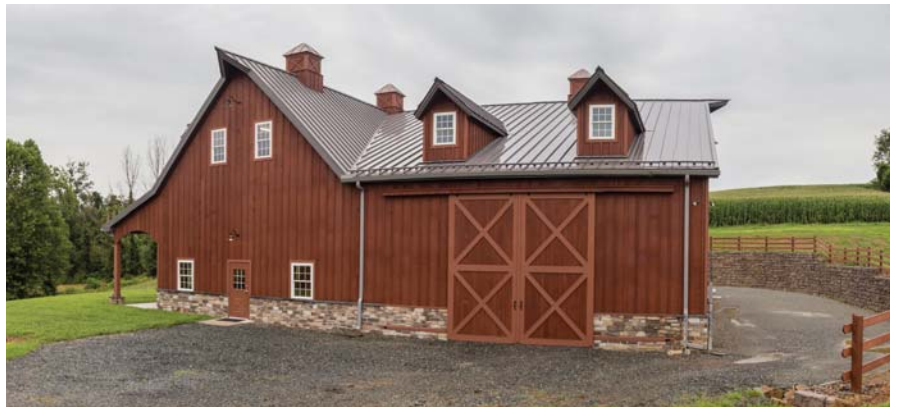
McElroy Metal panels top off this upscale board and batten barn. PHOTO COURTESY OF MCELROY METAL
