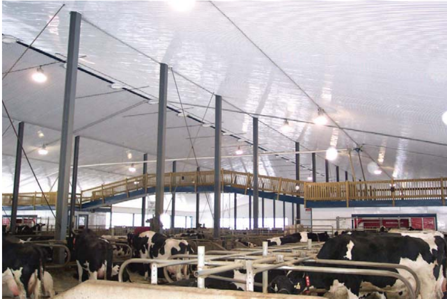
Palram's AG-TUF corrugated PVC liner panels are chemical-resistant, maintenance-free panels for interior cladding of agricultural structures. PHOTO COURTESY OF PALRAM
