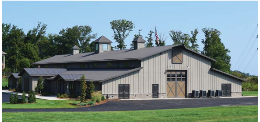
Graber Post Buildings has been supplying products and materials for horse barn construction since 1973. It also offers all sizes of tongue and groove lumber for stall construction. COURTESY OF GRABER POST BUILDINGS
