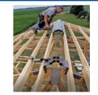
Ridgeline Safety Systems' fall arrest solutions make it easy for workers to tie off, thus preventing falls. The system has two main components: anchors and ridge hooks. Anchors attach to the trusses before setting or, for retrofits, as soon as the old ridge is removed. These permanent anchors provide immediate tie-off points and will be covered by the new ridge cap. Ridge Hooks are used after the ridge cap is on and provide nohole tie-off points for workers or repair technicians.
