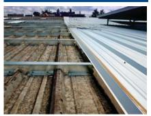
Roof Huggers are 10' long, tested, high strength, structurally correct, 16 gauge, 0.060" min., G-90, 50 KSI, "Z" shaped sub-purlins, specifically notched to let the ribs of any existing metal panel pass through the vertical leg of the "Z". This unique retrofit system allows any new metal roof to be installed over an existing metal roof without its removal, saving time and money, and allowing for thermal upgrading of the existing building.
