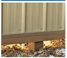
"Get" that all pressure-treated wood in ground contact will fail and that all "alternative" foundations are designed to "separate wood from ground contact." You'll "go" Post Protector! All the goodness of post frame... simplicity, speed, in-ground strength, DIY friendliness, and of course, value... just without the ground contact.
