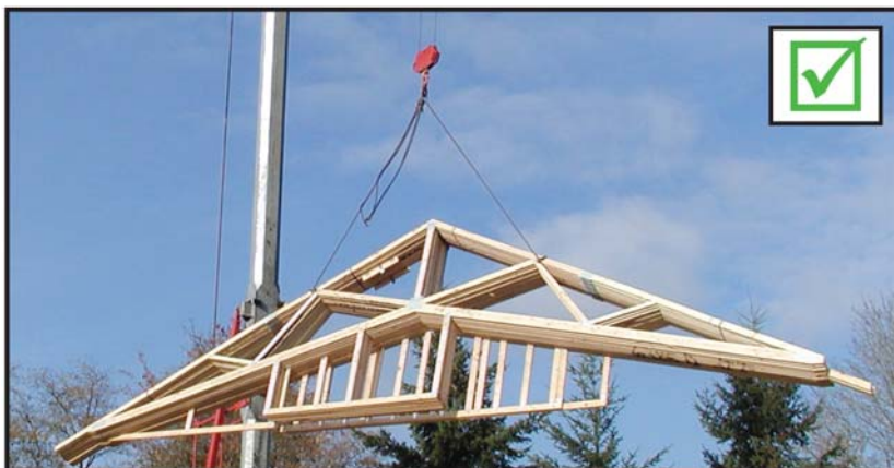
PHOTO B1-12: For trusses between 45-60 feet in length, at least two pick points should be used to lift a bundle. Photos courtesy of SBCA.
